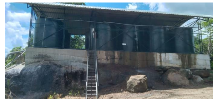
Lifted irrigation system at Siyambalanduwa
