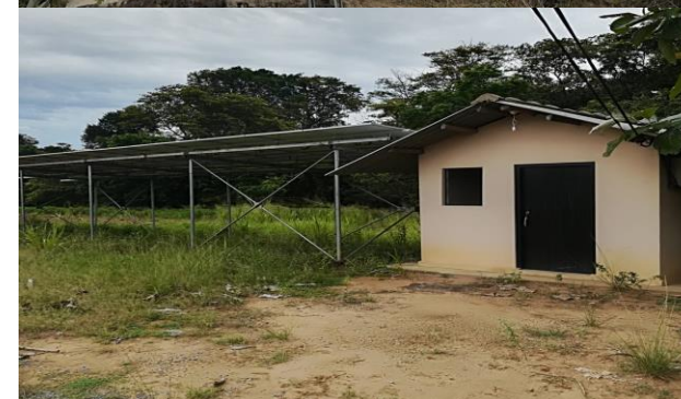
Lifted irrigation system at Bandiyawa, Madagama
