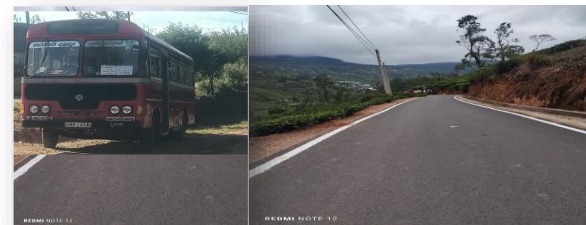
Improvement of Wakkadahinna Access Road.....
