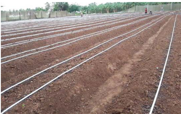
Figure 3: Drip Tapes lines installed.
