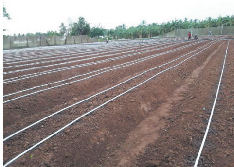
Figure 8: Drip Tape Installation
