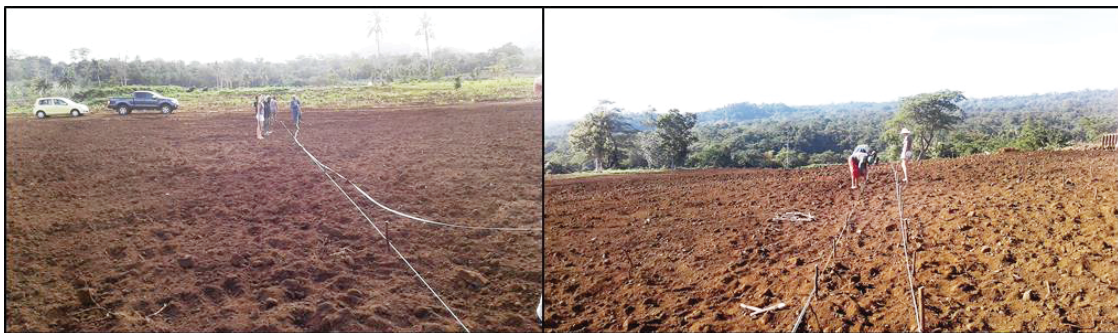
Laying Out the Base Line
