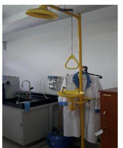
Figure 9: A shower installed at lab for safety purposes of the technical staff
