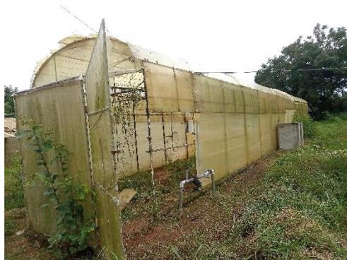
**Figure 4: A degraded polytunnel**
