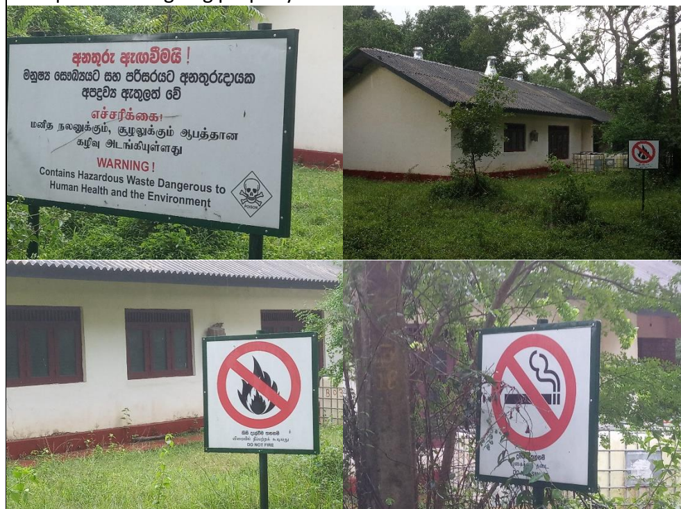
Figure 8: Chemical waste store located at Mahailuppallama research station
