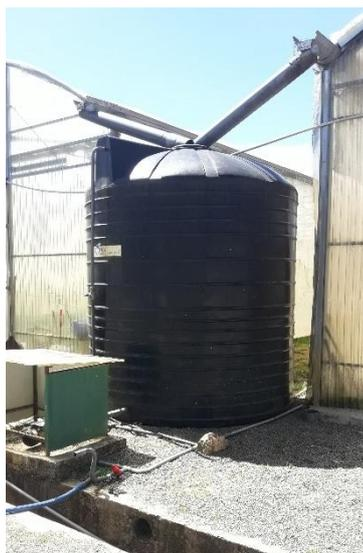
Figure 18: The rainwater harvesting system established
