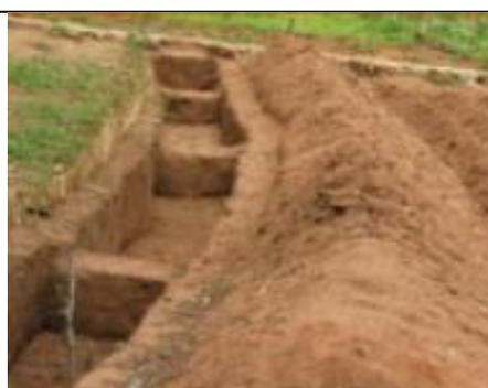
Figure 12: Newly constructed lock and spill drain
