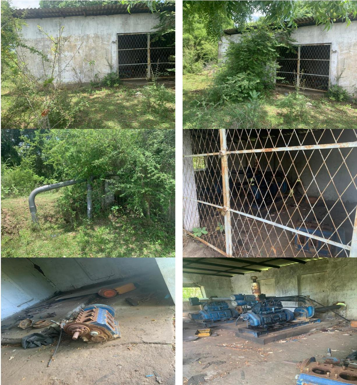
Figure 7: Photographs of existing damaged pump house
