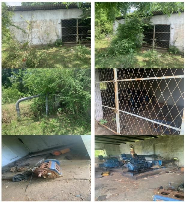
Figure 7: Photographs of existing damaged pump house
